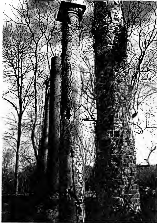
Figure 38: View of columns showing overgrowth of vines
